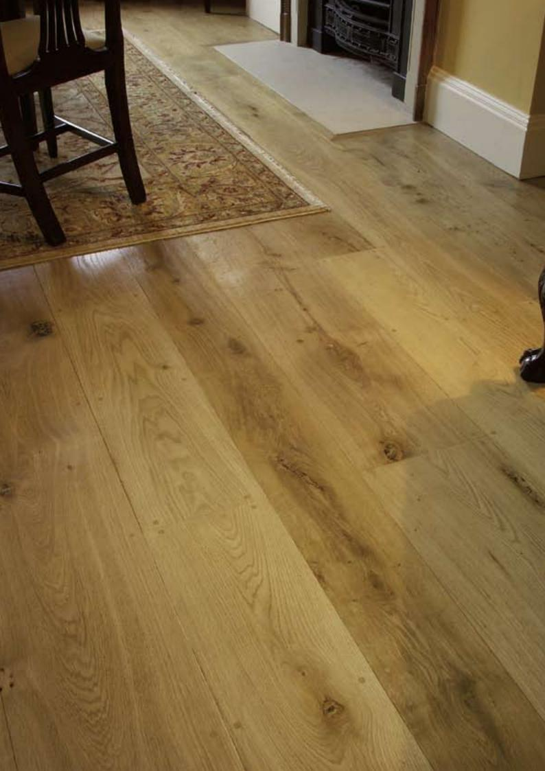
This hands-on approach applies to the preparation and installation of our reclaimed flooring as well. Reclaimed floor boards must be de-nailed in a laborious process that cannot be mechanised. Then, each board is prepared and sanded individually to retain the original patina of age.
