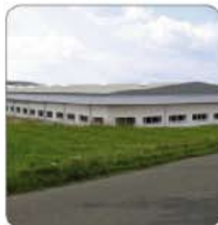
6. Markersdorf, Saxony Production of the buckles
