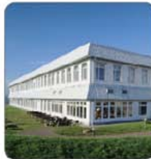
3. Asbach, Rhineland-Palatinate Form construction
